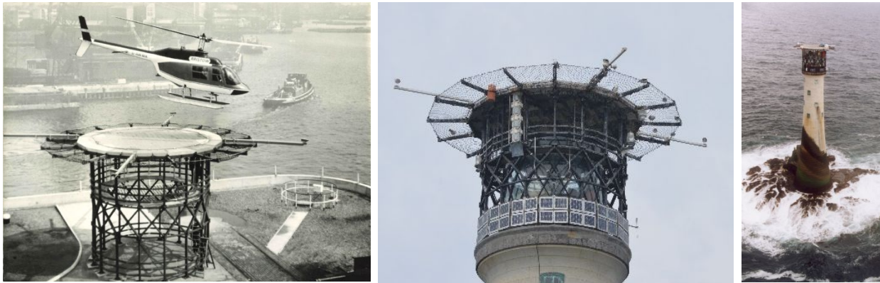
Figure 4. Wolf Rock helideck (a) trial at Trinity House's Blackwall depot (b) contemporary view (c) the 'new' vernacular of a helideck-mounted lighthouse.
