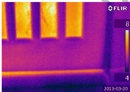
Fig 1 Thermal image showing a draught below the exterior door.
